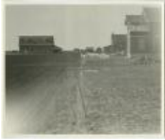
[The barn and some houses, Indian Residential School, Edmonton] (13d-c5704-d20)
