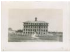
Norway House Indian Boarding School (13d-c5712-d29)
