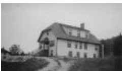
Hospital, Morley, Alberta (a034712)
