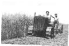
Harvesting operations, Alert Bay School (13a-c002177-d0066-001)
