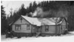
Preventorium, St. Michael's School, Alert Bay, BC (13a-c002177-d0065-001)
