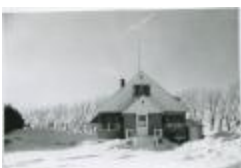
Principal's Residence (13d-c5713-d2)
