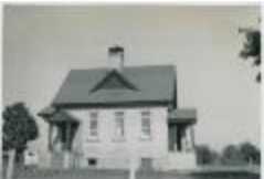
ONEIDA # 3 - One of the older schools. Continued in use. (13d-c5715-d45)
