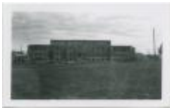
Norway House Indian Residential School : new building under construction (13d-c5712-d23)
