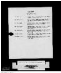
Cowichan Agency - Kuper Island Industrial School - Inspector Of Construction, 1914 (2057507)
