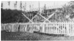
Alert Bay School - Principal building shack (13a-c004554-d0045-001)
