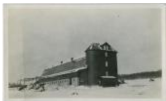
Dairy barn and silos, Brandon Institute (13d-c5711-d40)
