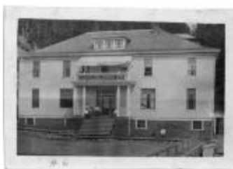
Elizabeth Long Memorial Home : before cement foundation (13d-c5703-d5)
