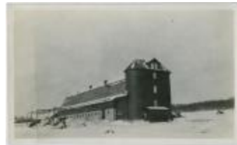
Dairy barn and silos, Brandon Institute (13d-c5711-d40)
