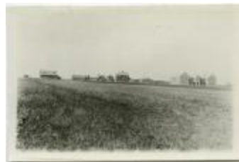
School buildings and campus, Indian Residential School, Edmonton, Alta. (13d-c5704-d21)
