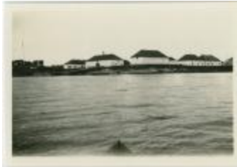
Hudson's Bay Company Fort, Norway House, Man. (13d-c5712-d62)
