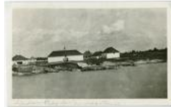
Hudson's Bay Company Fort, Norway House, Man. (13d-c5712-d75)
