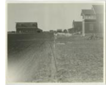
[The barn and some houses, Indian Residential School, Edmonton] (13d-c5704-d20)
