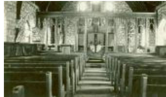
Chapel at Indian Residential School at Lytton (13a-c005010-d0004-001)
