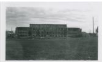
Norway House Indian Residential School : new building under construction (13d-c5712-d23)
