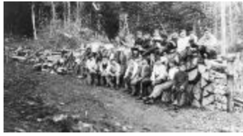
Alert Bay School Wood pacing crew - Job done! (13a-c004554-d0027-001)
