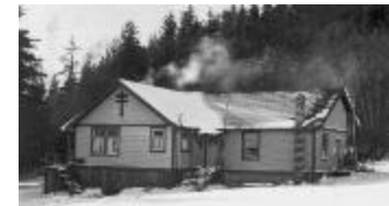
Preventorium, St. Michael's School, Alert Bay, BC (13a-c002177-d0065-001)
