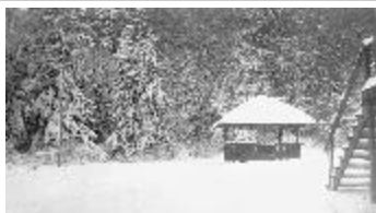
Alert Bay School, B.C. - Lots of snow behind preventorium (13a-c004554-d1081-001)
