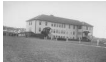
Morley Residential School after new wing was built (a034663)
