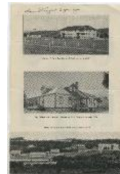
Morley Indian Residential School. rebuilt in 1935 (MOA_20180215_001)
