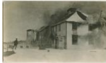
Norway House Indian Boarding School on fire (13d-c5712-d38)
