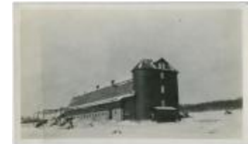
Dairy barn and silos, Brandon Institute (13d-c5711-d40)
