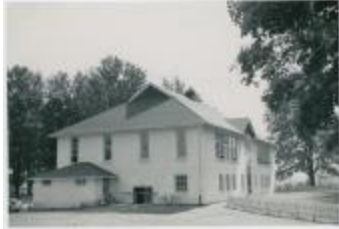
NEW SCHOOL, viewed from the south. Not occupied until January 17, 1949. (13d- c5715-d46)
