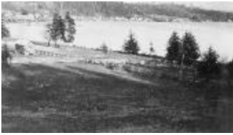
Alert Bay from behind Boy's School - Principal's shed and part of orchard in foreground (13a-c004554-d0006-001)
