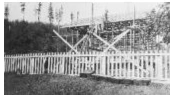
Alert Bay School - Principal building shack (13a-c004554-d0045-001)
