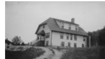
Hospital, Morley, Alberta (a034712)
