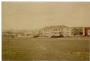
2-room day school, Residential s[school], New Day School [Morley Residential School] (13d-c5705-d2)
