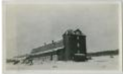
Dairy barn and silos, Brandon Institute (13d-c5711-d40)
