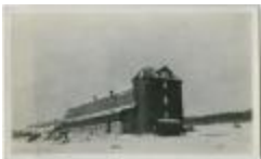
Dairy barn and silos, Brandon Institute (13d-c5711-d40)
