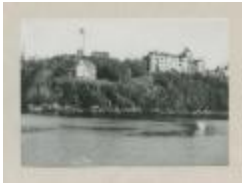
[Alberni?] Residential School (38f-c000591-d0001-002)
