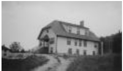
Hospital, Morley, Alberta (a034712)
