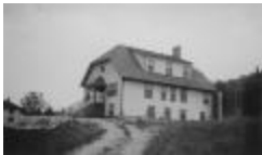
Hospital, Morley, Alberta (a034712)
