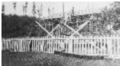
Alert Bay School - Principal building shack (13a-c004554-d0045-001)
