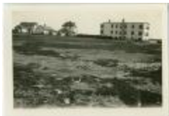
[Hospital run by the government, Norway House, Man.] (13d-c5712-d65)
