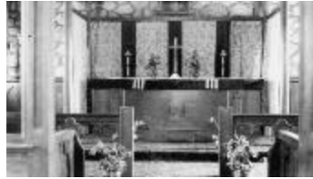
St. George's Church - Interior, Lytton, B.C. (13a-c004554-d1040-001)
