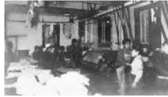
Alert Bay School - Laundry Room (13a-c004554-d0078-001)
