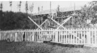
Alert Bay School - Principal building shack (13a-c004554-d0045-001)
