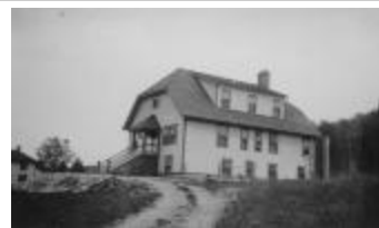
Hospital, Morley, Alberta (a034712)
