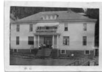
Elizabeth Long Memorial Home : before cement foundation (13d-c5703-d5)
