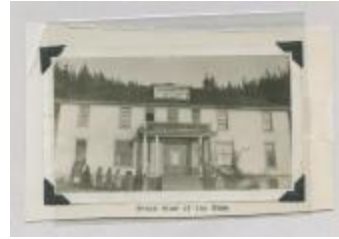
Front View of Home (38f-c000134-d0001-001)
