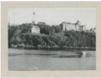
[Alberni?] Residential School (38f-c000591-d0001-002)
