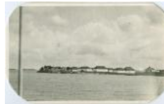
[Hudson's Bay Company Fort, Norway House] (13d-c5712-d76)
